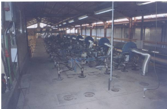
Fig. 12 Overview of the roof burners.
