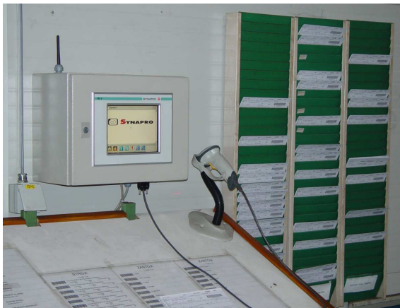
Fig. 1 Example of information terminal (manufactured by Synatec).
